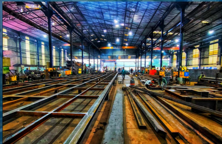
Heater Panel Numaligarh Oil Refinery
